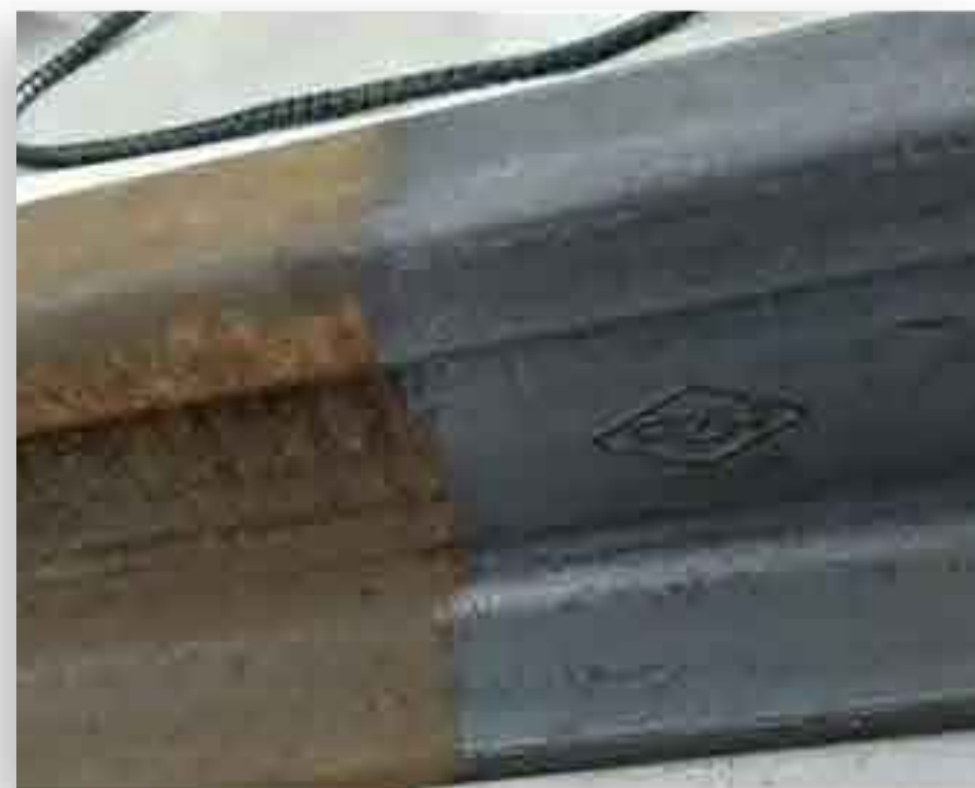
Track rust removal and cleaning
